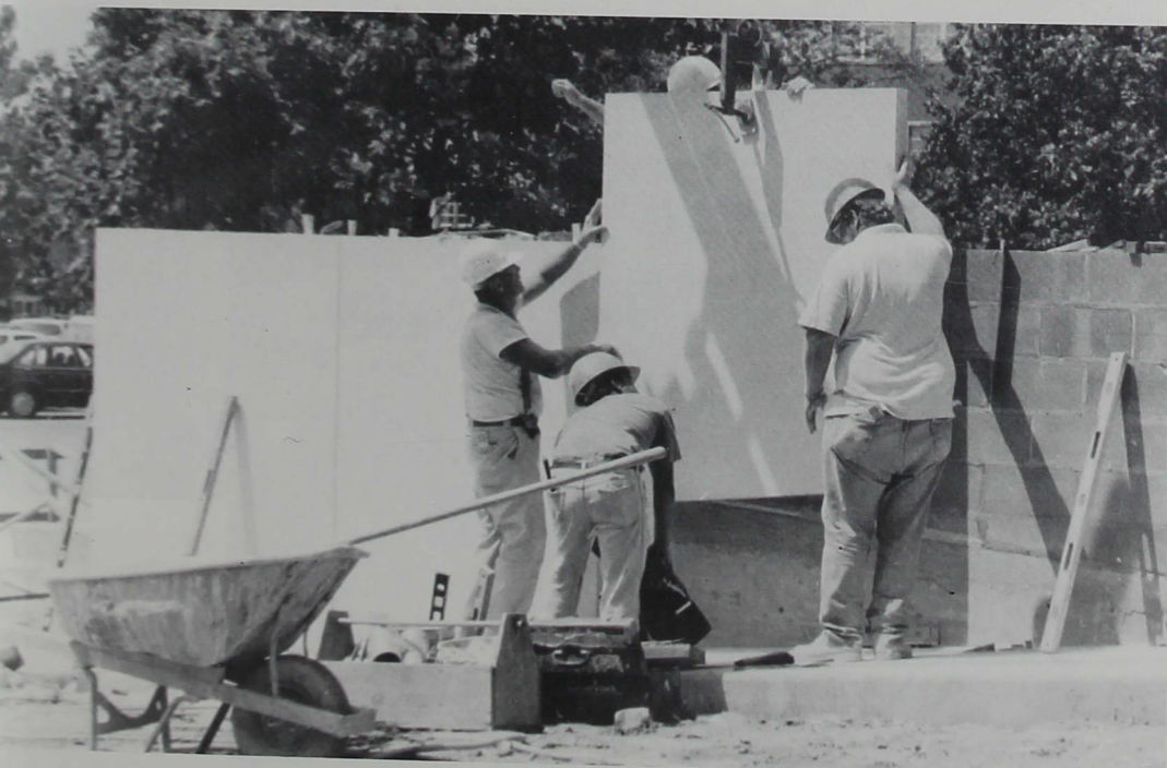
Above: Construction workers place the stone slabs that form the handicapped ramp in Schwitzer Center. An elevator was also added to Schwitzer to aid accessibility.
